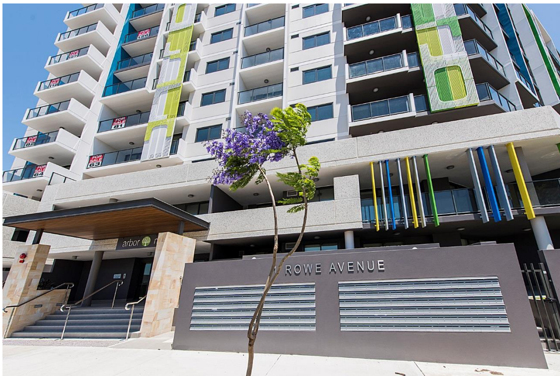
Above Images: Completed – Arbor North
