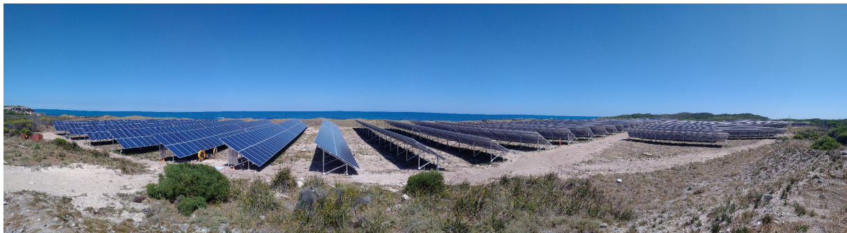
Garden Island Microgrid 2MW solar farm construction
