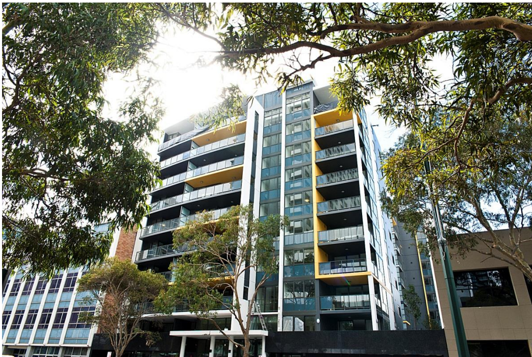
Above: Adelaide Terrace frontage of Au project.
