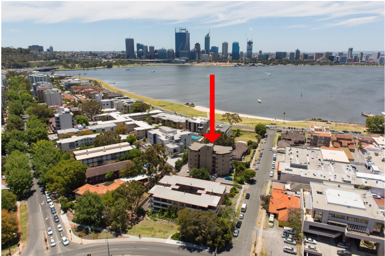
Above: The location of 5-7 Harper Terrace South Perth and the existing buildings.
