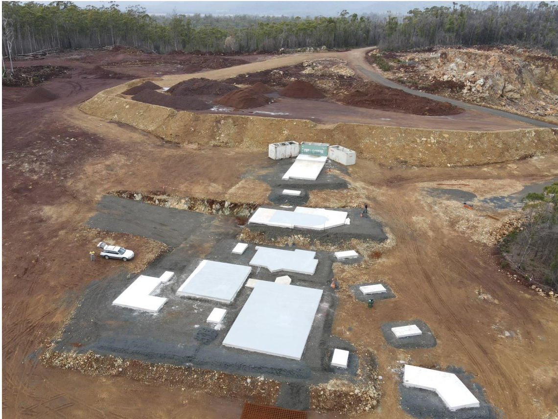
Figure 2 | Wet Screening Plant Site 19th January 2021
