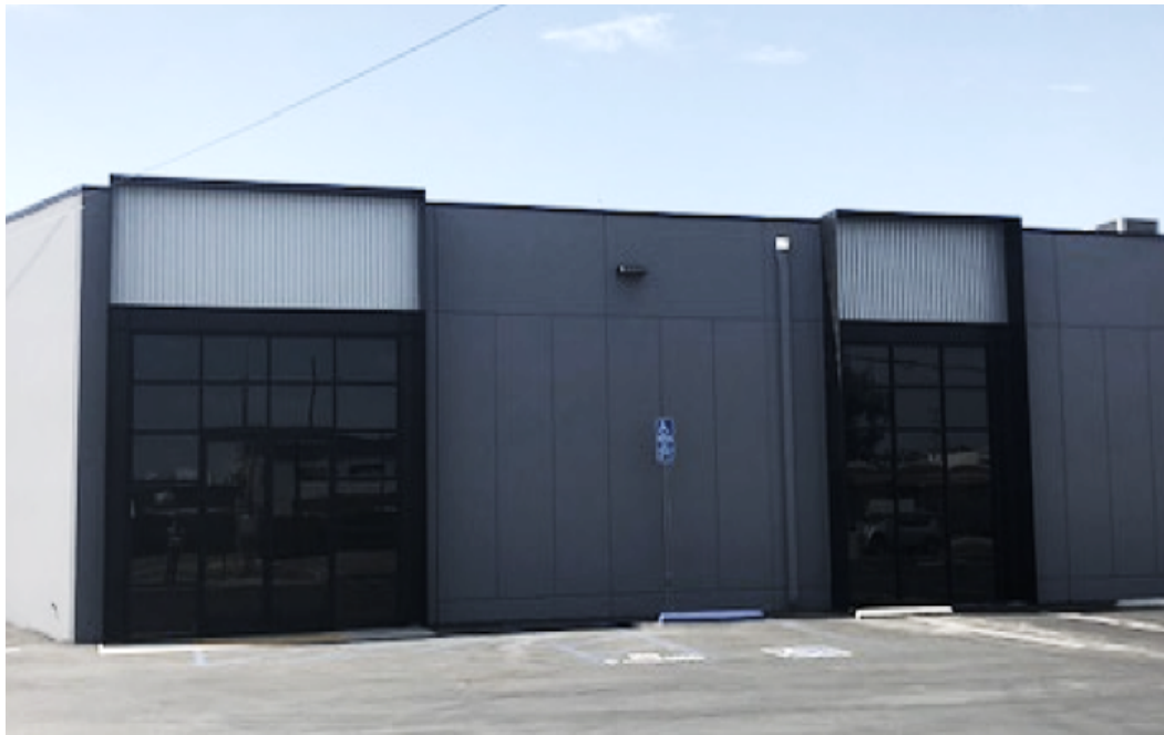
Amaero USA Facility in Los Angeles, California
