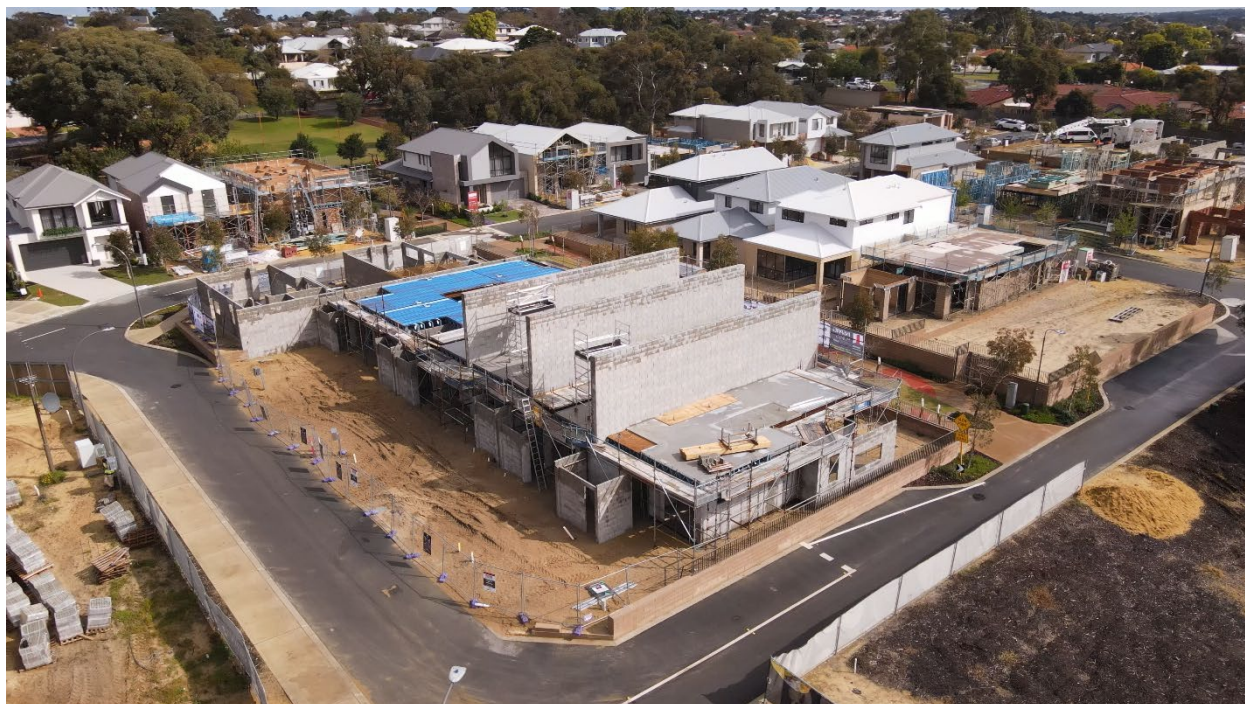
Drone image of Willagee construction site showing completion of upper floors
