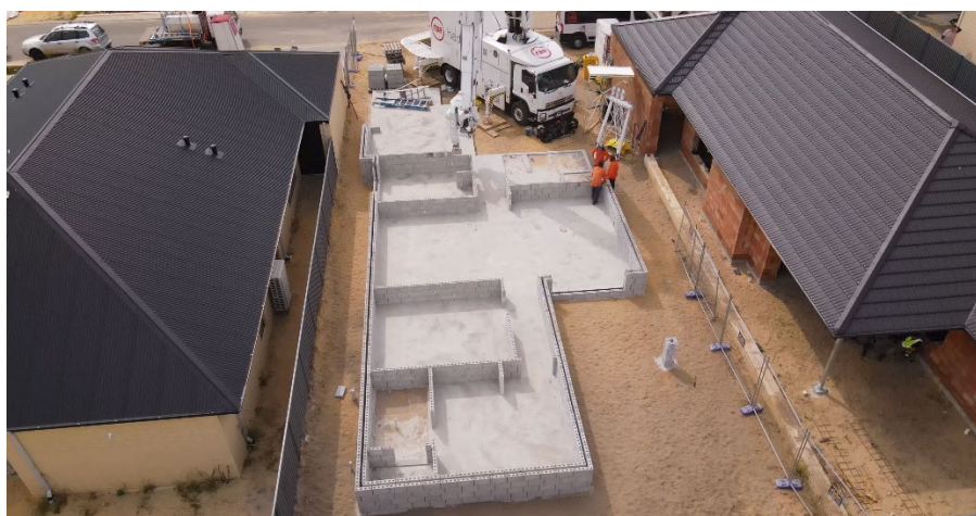
Final home in the Wellard portfolio under construction
