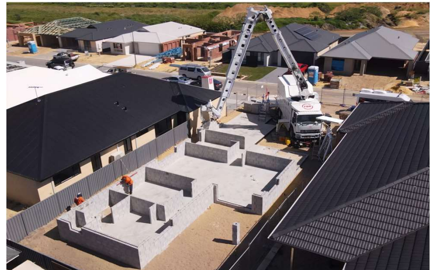
Hadrian X® building a structure in Perth, generating zero on-site masonry waste
