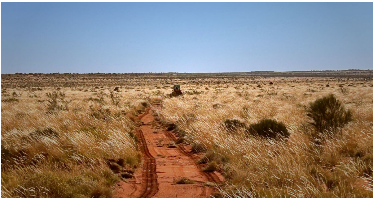
Figure 1: Access track construction at the Madman Project, Little Sandy Desert WA, May 2026
