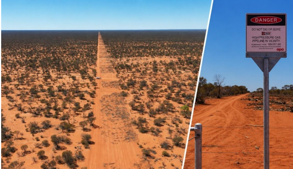
Figure 7: Existing high-pressure gas pipeline infrastructure in the vicinity of the Jupiter Project.
