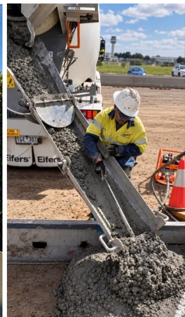
Eifers concrete incorporating G360's MKX calcined clay at Melbourne Airport Business Park and a pavement pour at Melbourne Airport.
