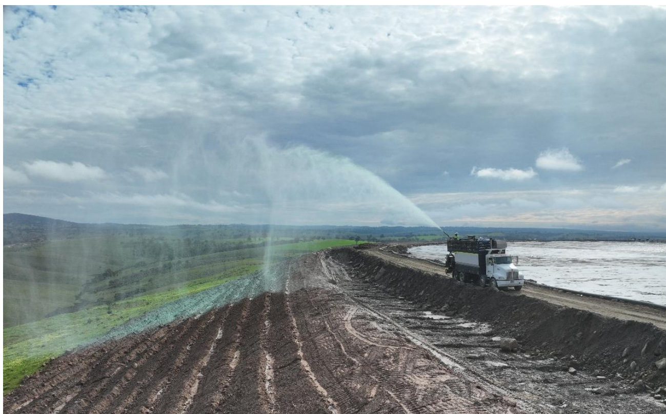
Figure 1: Hydroseeding of the Kanmantoo TSF embankment as part of Kantra's progressive rehabilitation program
