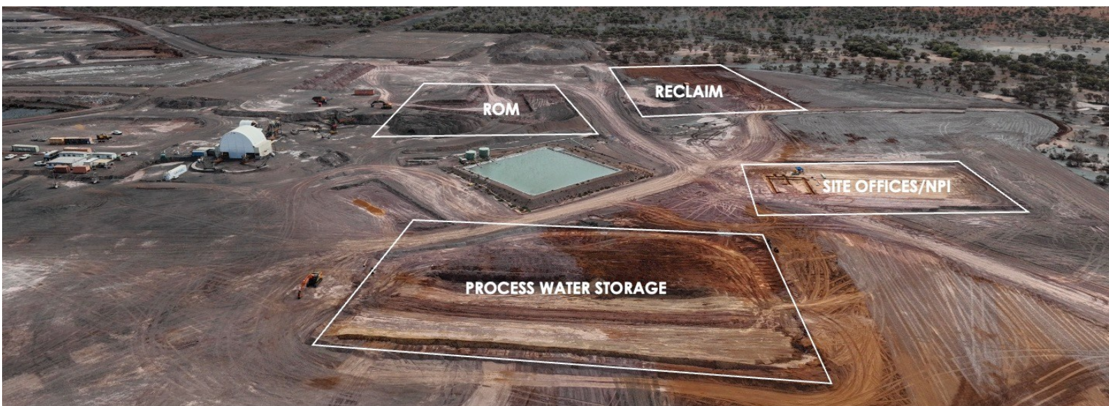
Figure 1: Aerial overview of early works activities at the Butcherbird Project.
