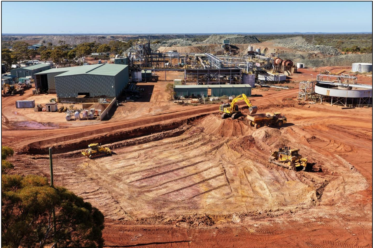
Figure 3 – BSPH – Earthworks underway in the Processing area
