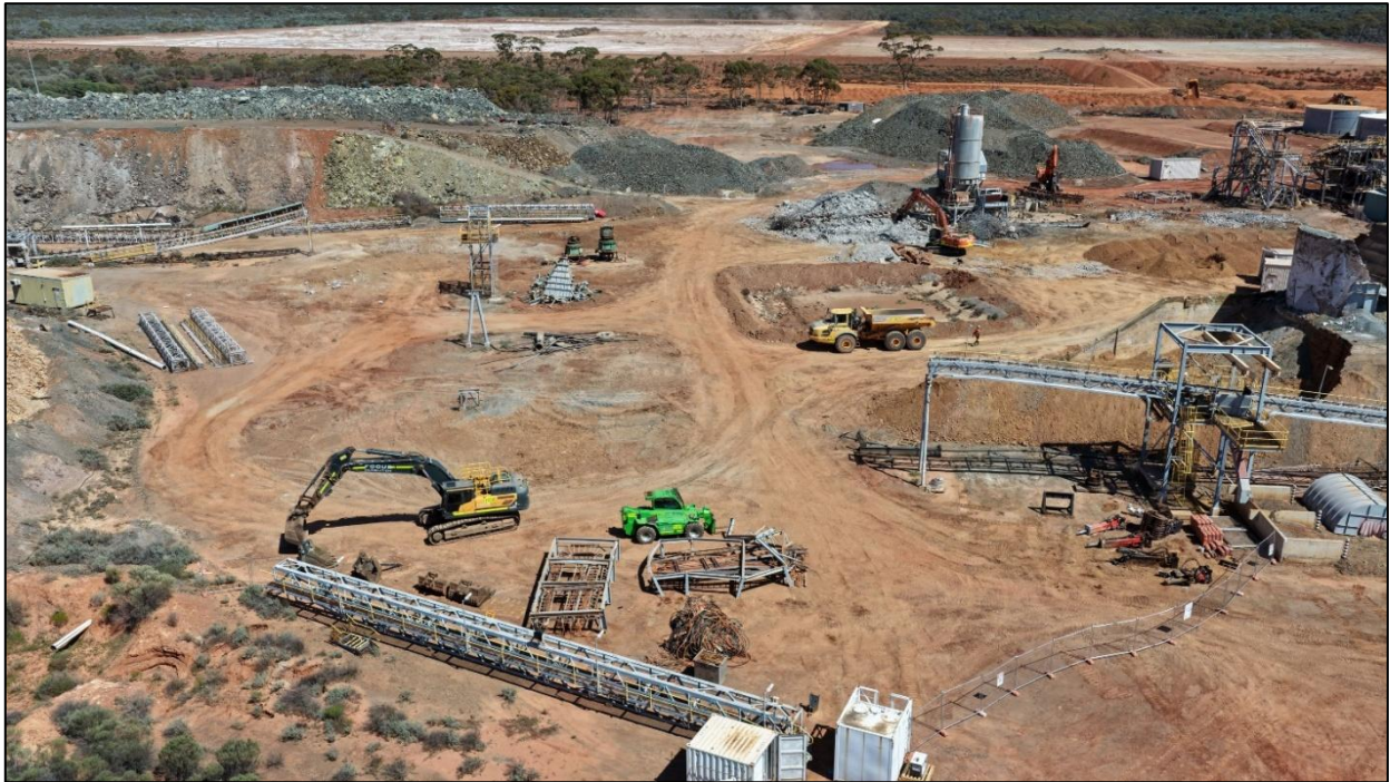
Figure 2 – BSPH – demolition of redundant conveyors and structures
