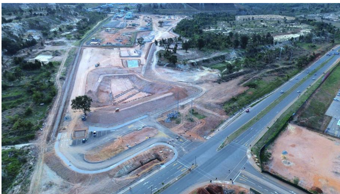
IMAGE 3: ACCESS ROADS AND POLLUTION CONTROL DAM UNDER CONSTRUCTION
