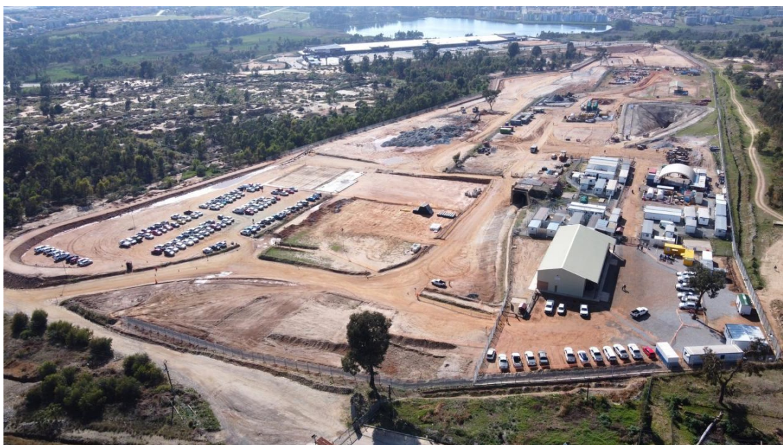
IMAGE 1: AERIAL VIEW OF QALA SHALLOWS SHOWING THE DECLINE PORTAL, WORKSHOP, SITE OFFICES AND SURFACE INFRASTRUCTURE WORKS
