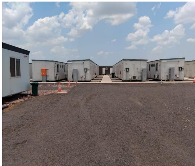
Figure 10: Camp Accommodation Buildings
