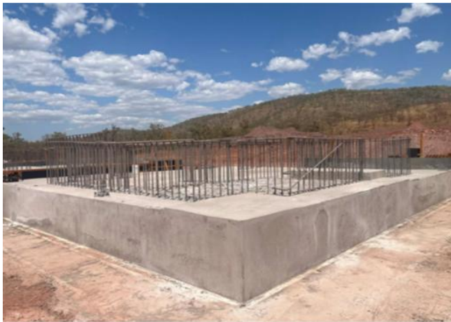
Figure 3: Mill Foundations at Sorby Hills
