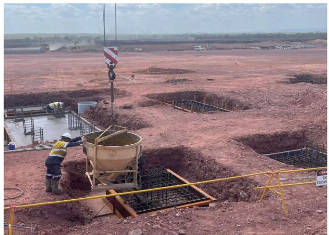
Figure 4: Floatation Area Footings
