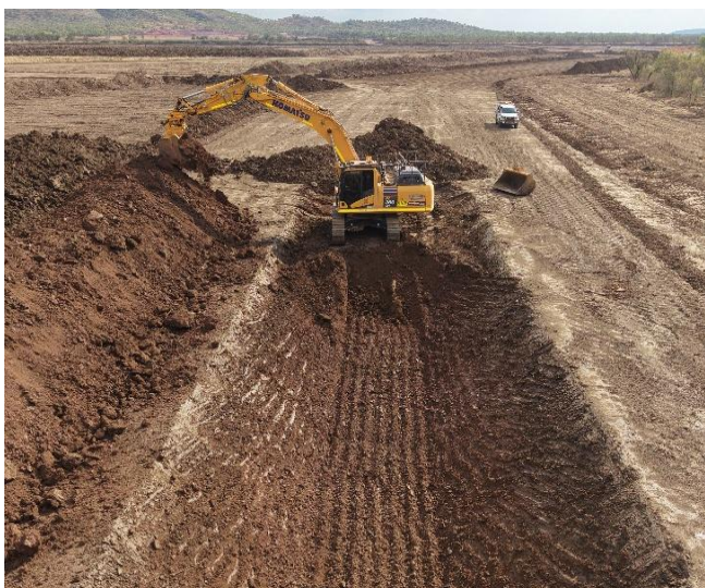
Figure 7: Key Way Excavation – Evaporation Pond
