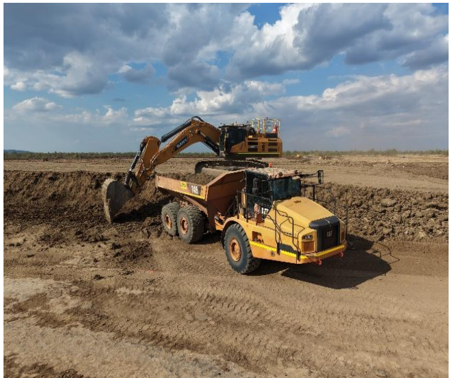
Figure 8: Topsoil Removal
