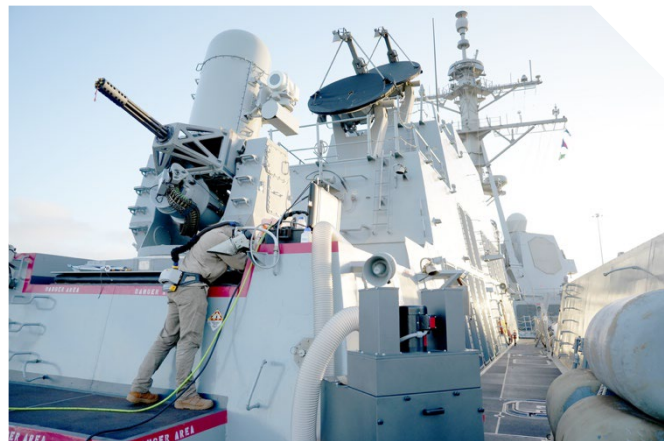
Technician repairing corrosion on the deck of the USS Momsen (DDG-92) with the TKF™ Tactical System
