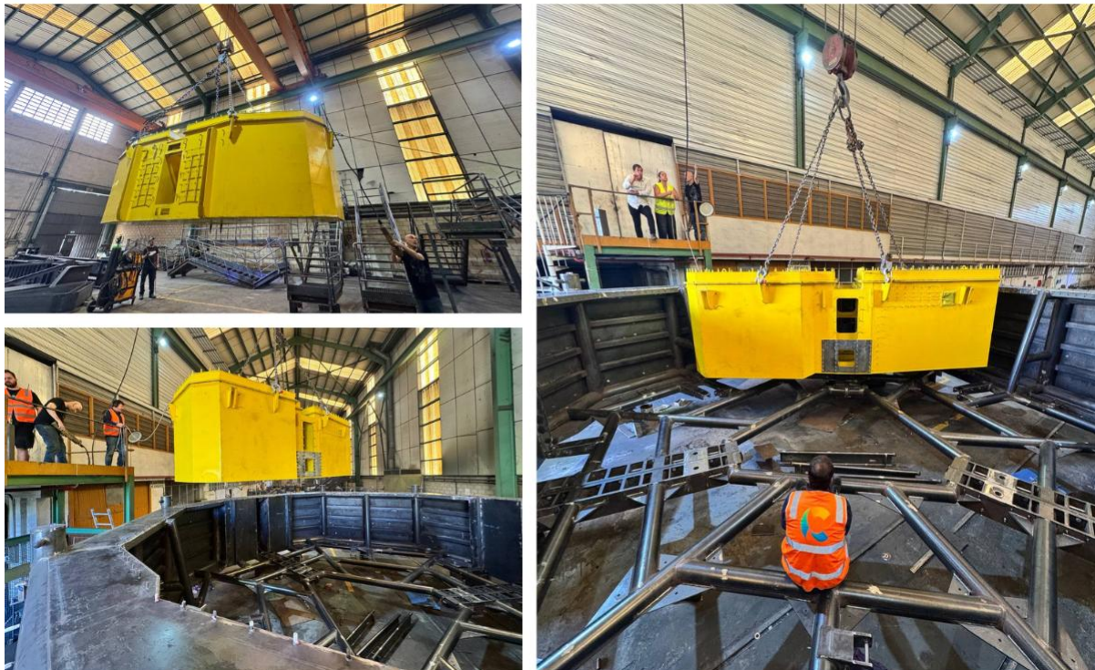
PTO (yellow module) and Buoyant Actuator (BA) fit testing
