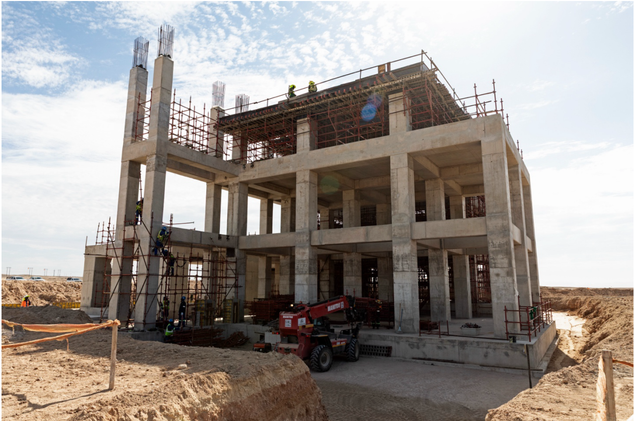
Figure 4: Side view of the secondary and tertiary crusher facility
