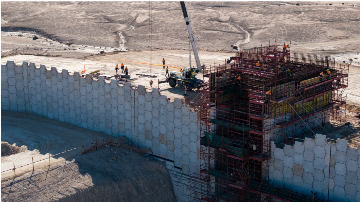
Figure 1: The primary crusher concrete structure is being advanced concurrently with the pre-cast retaining wall installation
