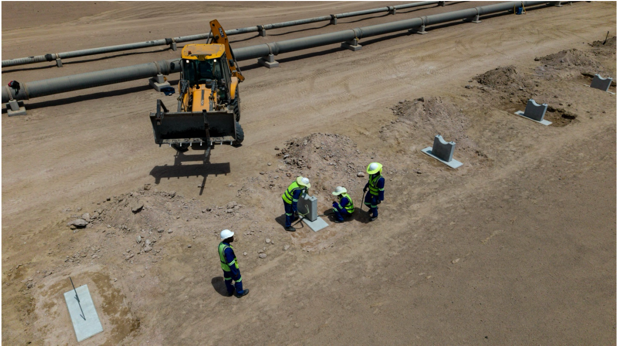
Figure 5: Permanent pipeline pipe pedestal installation.
