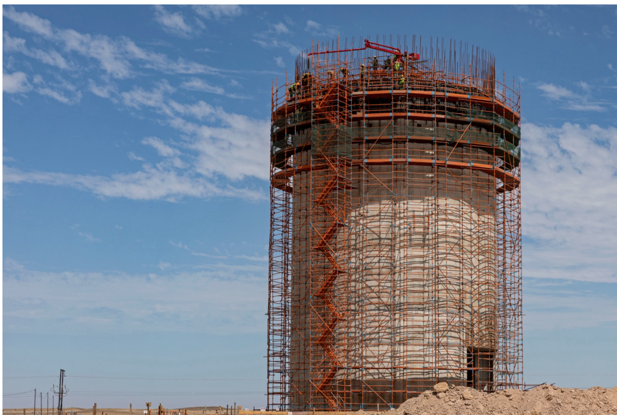
Figure 3: Ground level view of fine ore silo.
