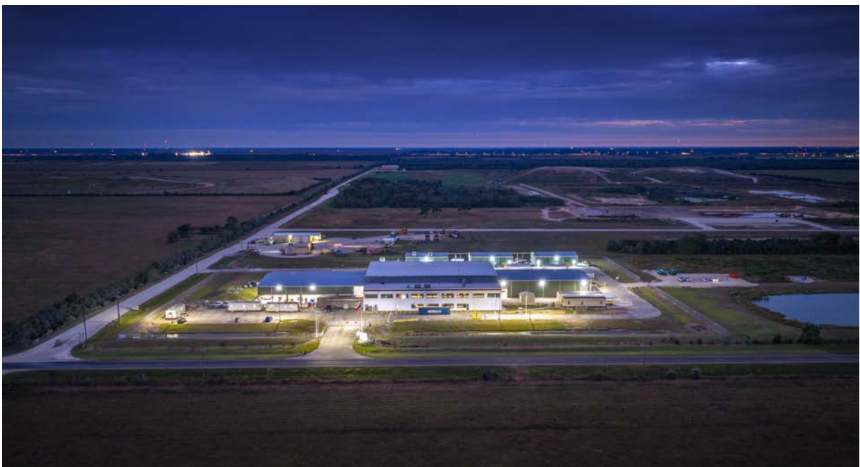
Figure 3: Aerial view of Gator Point and its supporting infrastructure. 21 October 2026,
