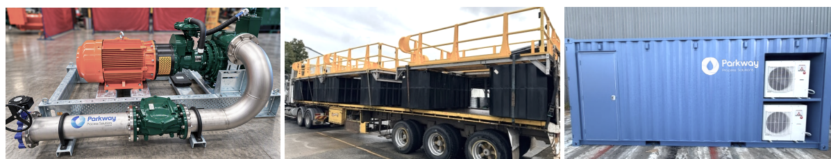
(i) Fabrication of specialised pump skids (1 of 6). (ii) Transport of pump pontoons for mine pit water. (iii) Fabrication of VSD equipment controls (1 of 2).
