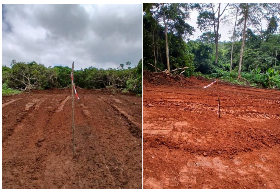
Figure 2. RC pad preparation at the Bondoukou Gold Ridge Project during the quarter.
