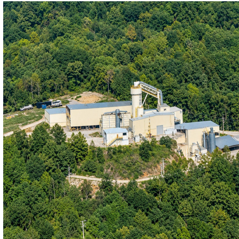
NewCarbon Processing plant, Inez, Kentucky (October 2026)
