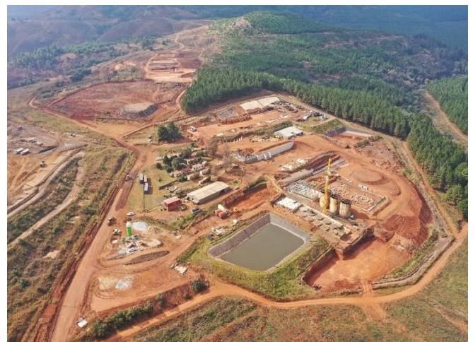
Figure 6: Site aerial view highlighting plant footprint
