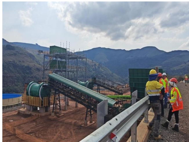
Figure 8: Team observation of conveyors
