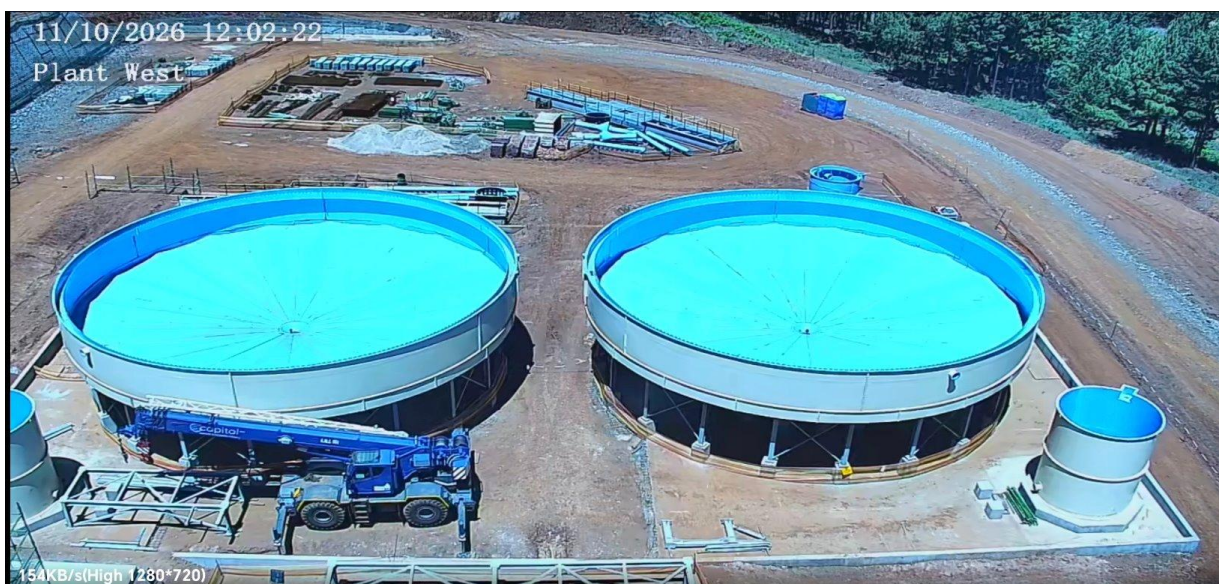
Figure 11: Thickener tanks installed at site
