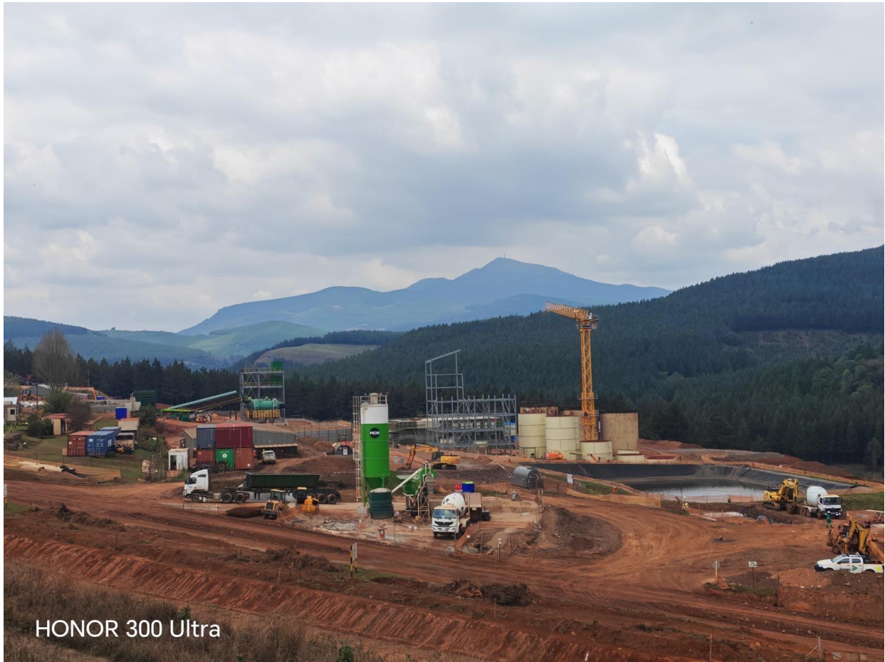
Figure 22: TGME Plant construction progress including on-site batch plant
