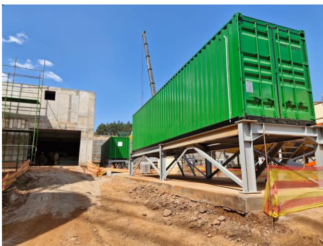
Figure 9: Gold Room construction and MCC installation
