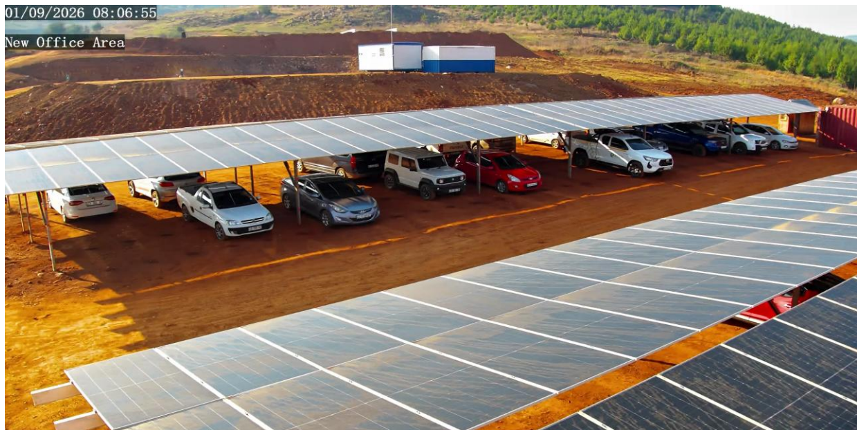
Figure 15: Construction of new employee parking facilities with solar roof panels generating 160 Kilowatts
