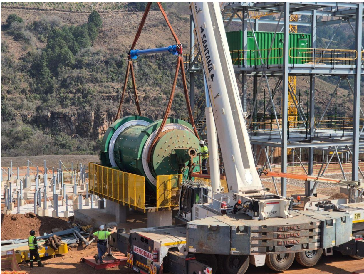
Figure 16: Installation of Twin Ball Mills
