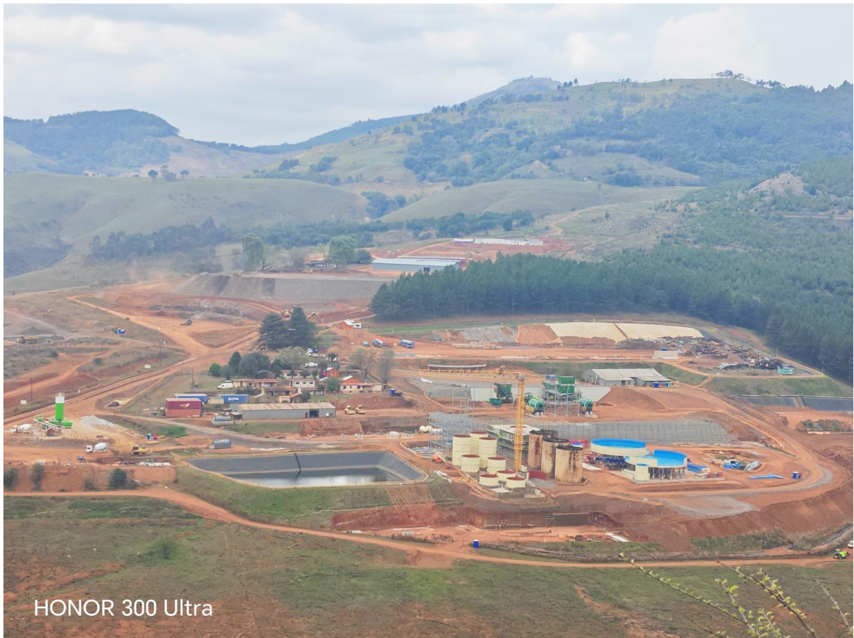
Figure 1: Aerial view of site construction with stockpile material in background to feed the plant
