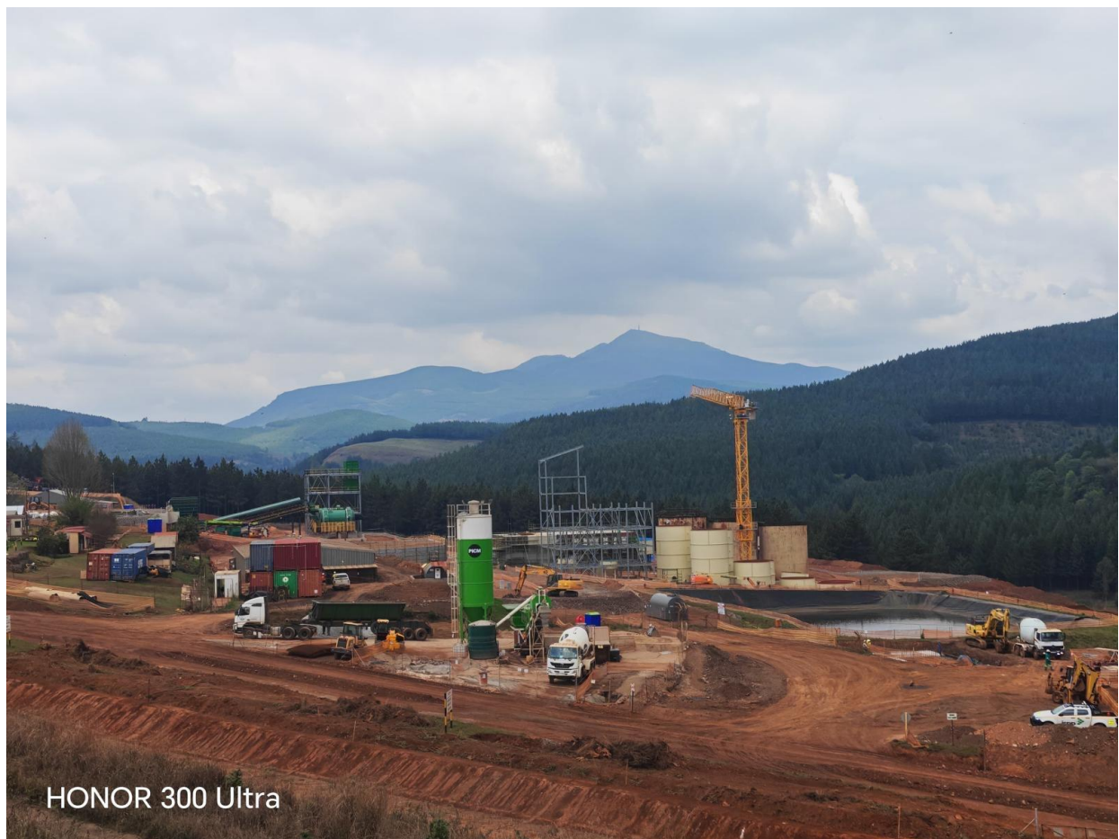
Figure 12: Concrete Pumping – Gold Room
