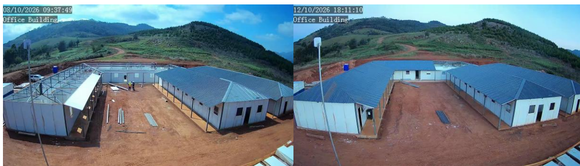
Figure 18: Offices and Administration Complex in progress
