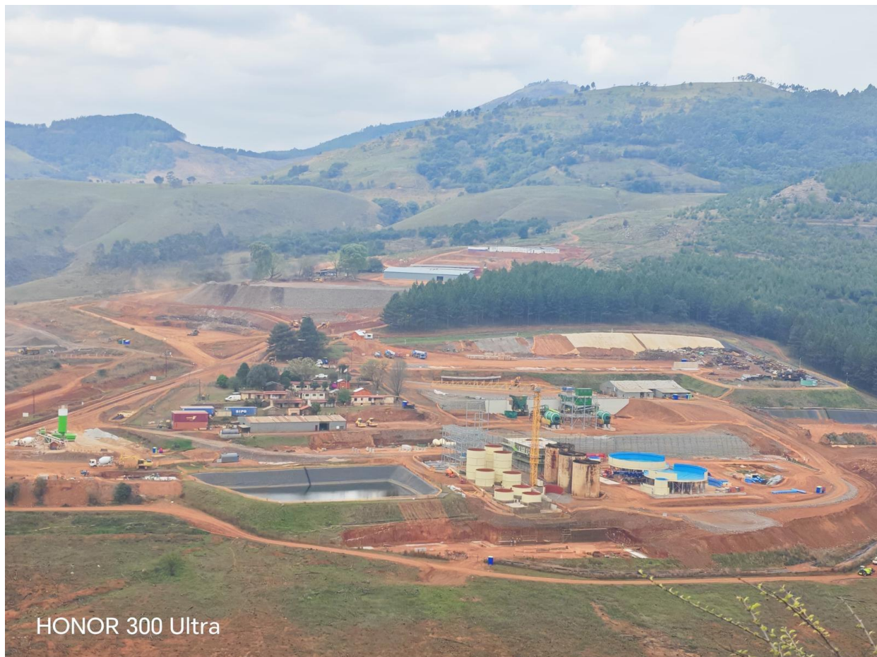
Figure 13: Thickener Tank foundations in progress
