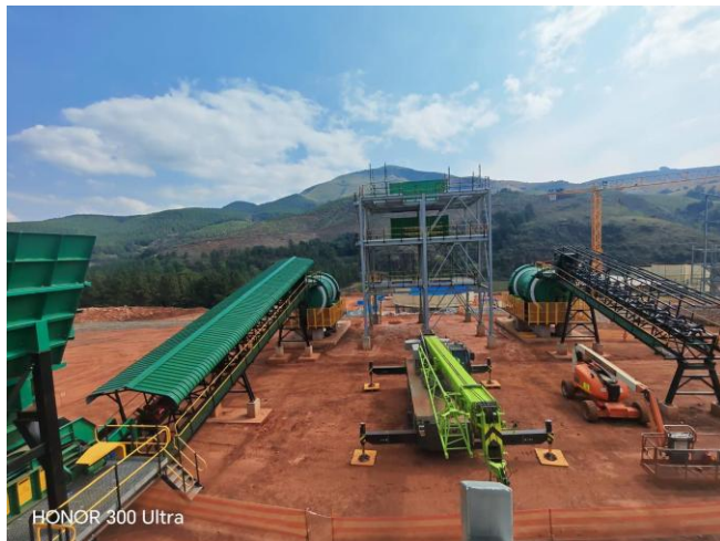
Figure 7: Installation of conveyors to feed ball mills
