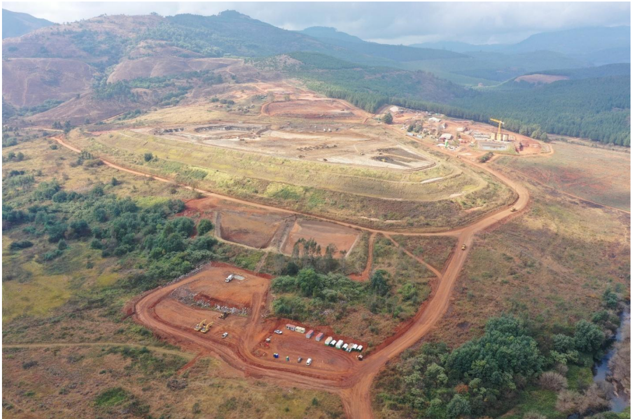
Figure 4: TGME Gold Project aerial view of the TSF (bottom: Laydown area; middle: TSF; top right: new plant under construction)
