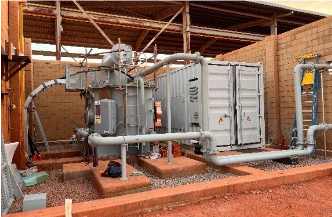
Rectifier installed
