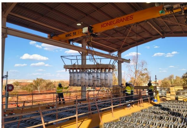
Installing anodes
