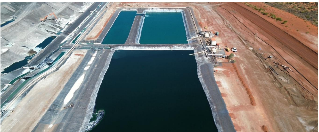
Arial view of ponds and W-drains
