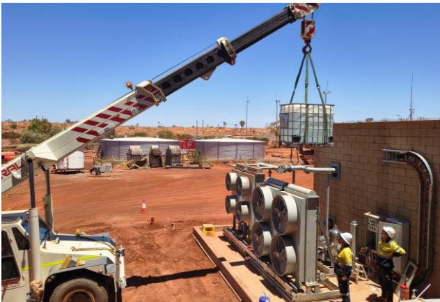
Filling of rectifier cooling circuit with demineralised water
