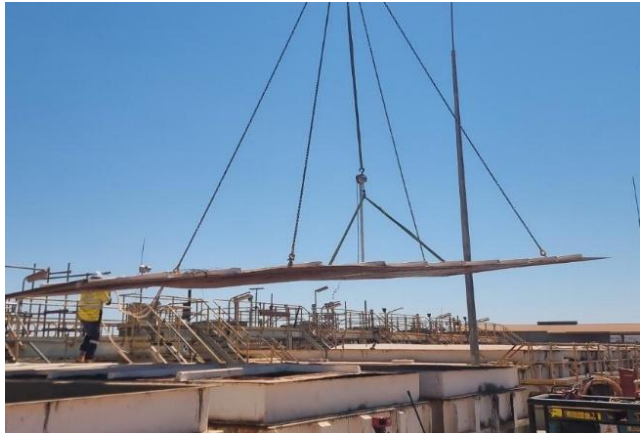
Settler tank lids lifted into place
