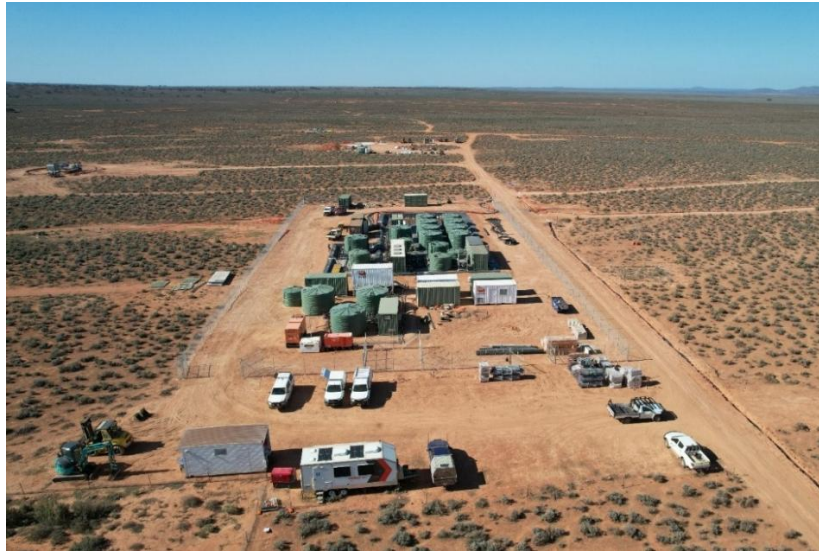
Figure 3: Samphire Field Recovery Trial plant in full operation (looking north)
