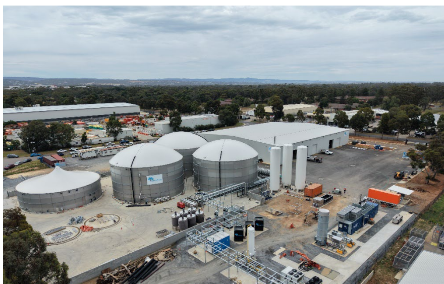
Image 2: SA1 Bioenergy Project Construction
