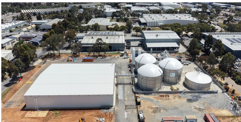
Image 1: SA1 Bioenergy Project Construction
