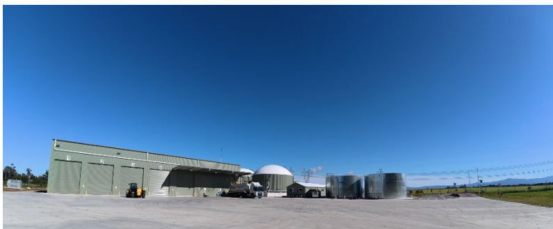
Image 10: Yarra Valley Water Lilydale Bioenergy
