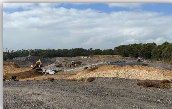
Image 8: Horsley Park Site Works
