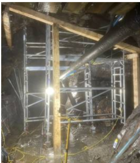
Figure 2: Cabin under construction at Llechfraith Adit Level
