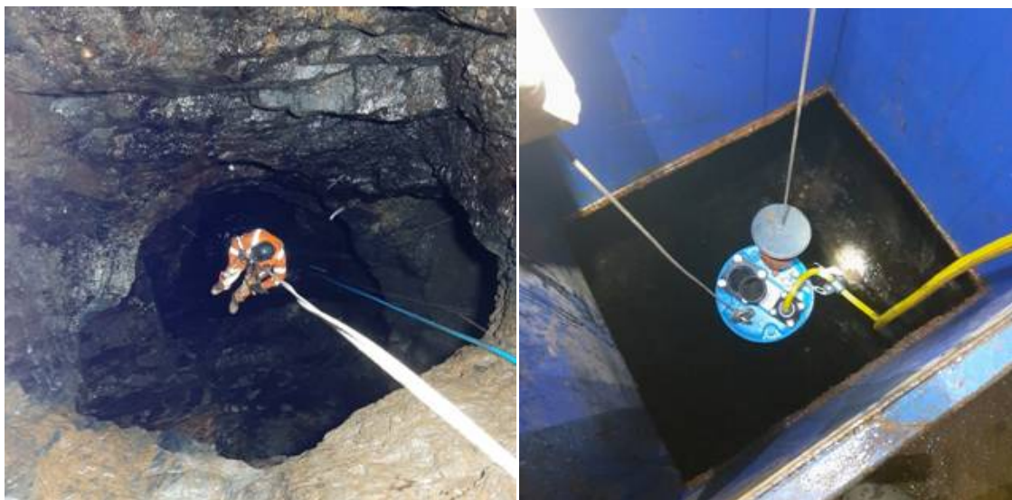
Figure 1: (left) personnel from Alba's underground works contractor inspecting Llechfraith Shaft; (right) new sludge pump being lowered to No.4 Level
