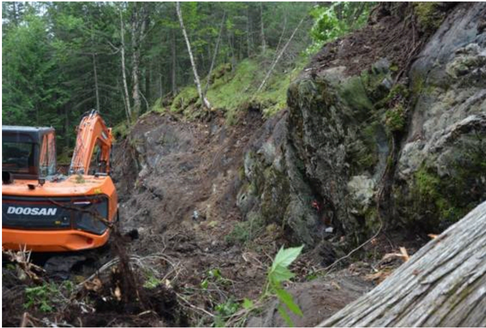
Figure 3 initial stages of 'stripping': mechanical removal of overburden
